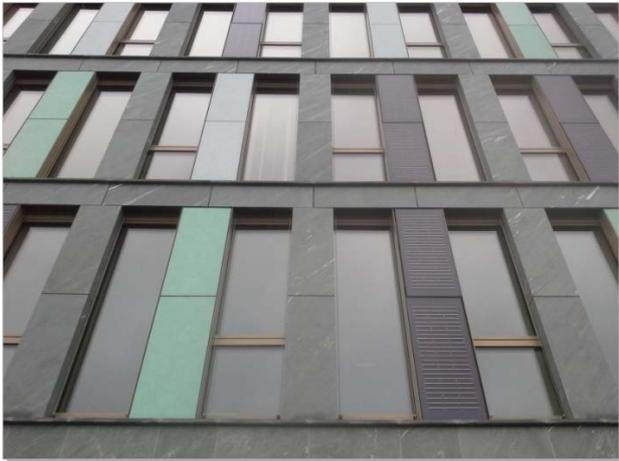
Figure 7. PV Modules in the Façade
